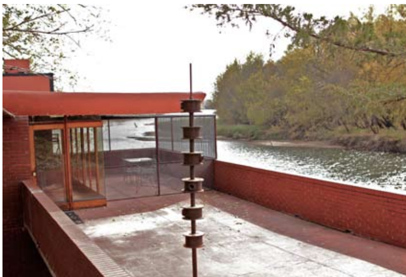
Above: the boathouse or “River Pavilion”, as Wright called it, on the Wapsipinicon River
